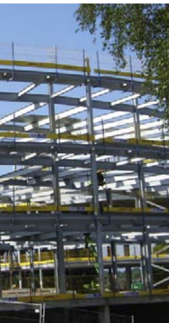
Below: A steel frame was chosen for its speed of construction.
